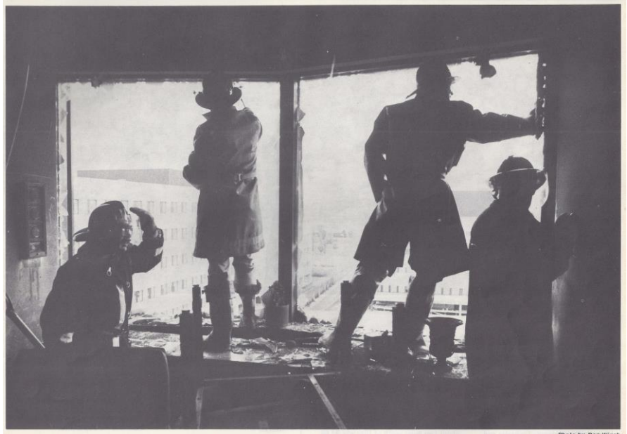
The fire in 3M's main administration building, Building 220, occurred in the early morning hours of July 25. Fire fighters from Maplewood, St. Paul and surrounding suburbs responded quickly to the call. Above, fire fighters work in an office in the badly-charred sixth floor after extinguishing the fire. Below, broken windows in the building give no clue to the kind of damage to the inside offices (lower right) that occurred.
