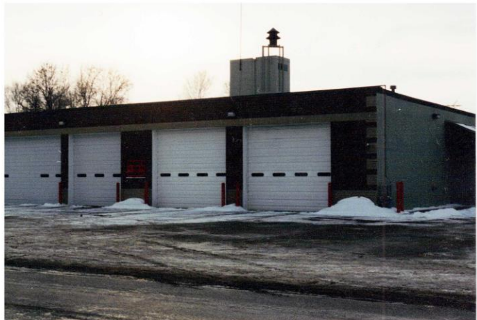
Parkside Fire Department 2001 McMenemy Street Maplewood
