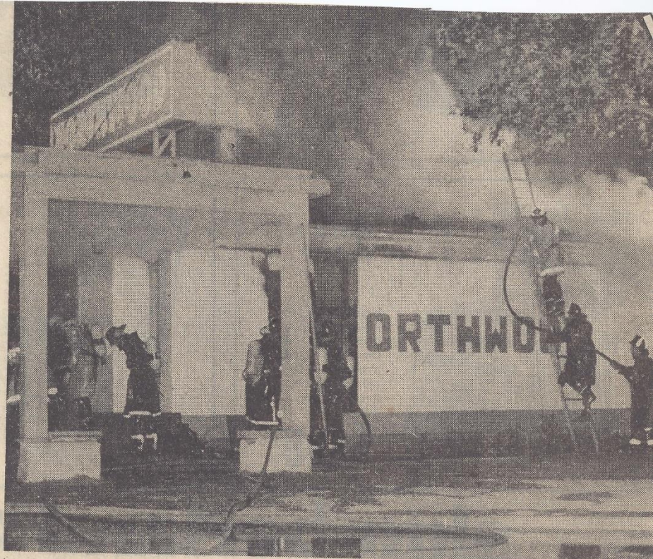
Firemen battling a blaze that destroyed the Northwood Country Club are shown as they worked through the night to try to save the building and keep the fire from spreading to a nearby nursing home.—Photo for the Dispatch by Dave Bade
